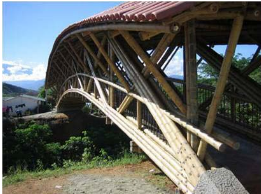
Fig.8: Puente 30m, Antioquia, J.Stamm
